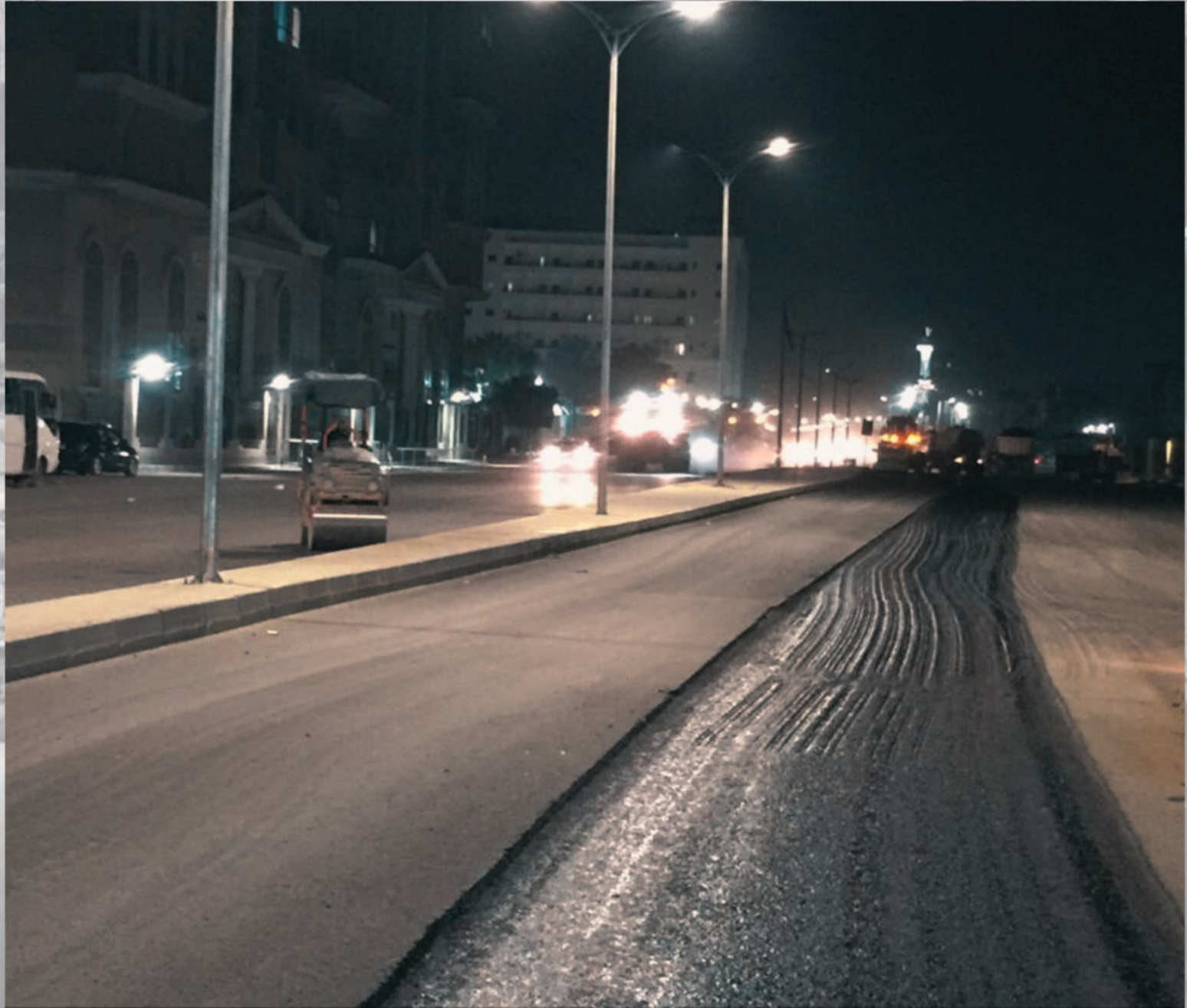
7 ROAD WORKS OVER A DISTANCE OF KM
